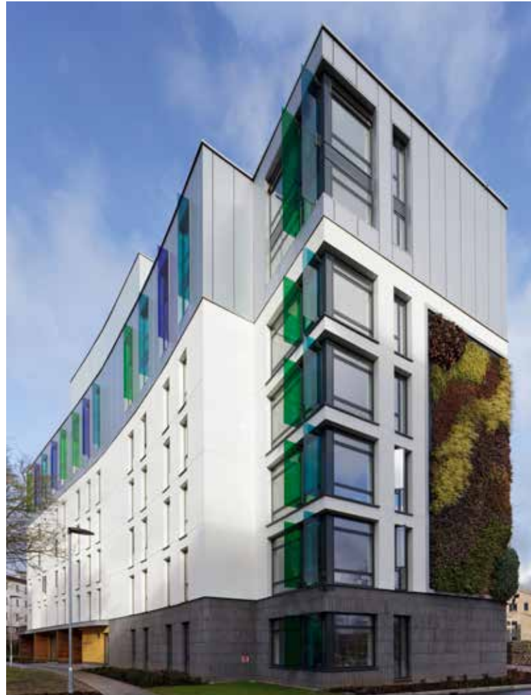
Crome Court, University of East Anglia, stores 1,226 tonnes of carbon in its timber superstructure.
